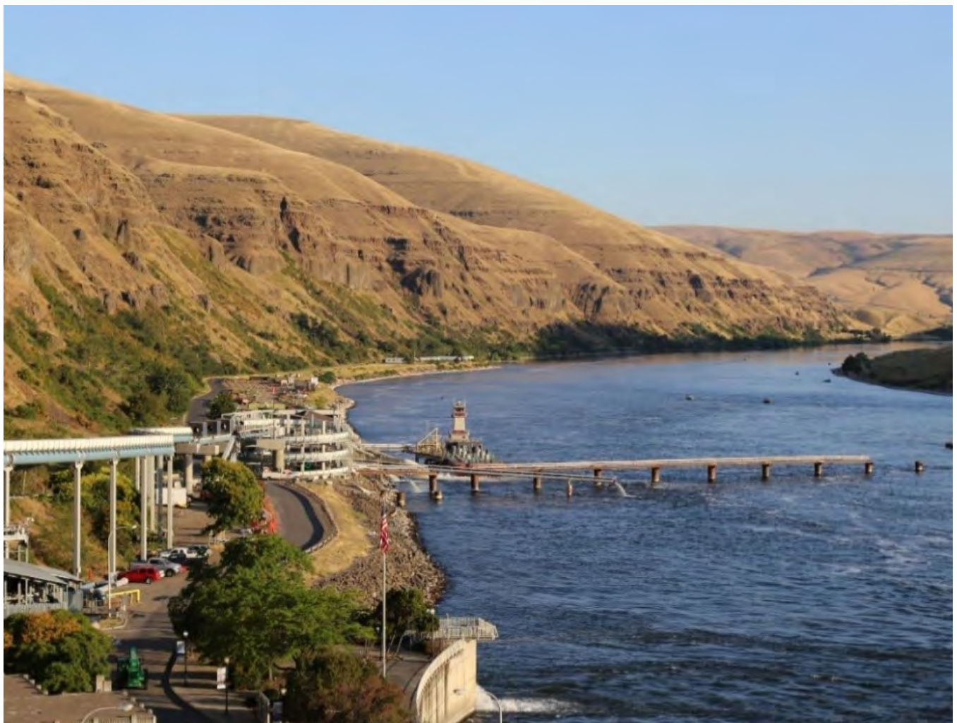
Figure 1-5. Lower Granite Dam New Juvenile Fish Facility, Bypass Pipe, and Fish Transportation Barge
