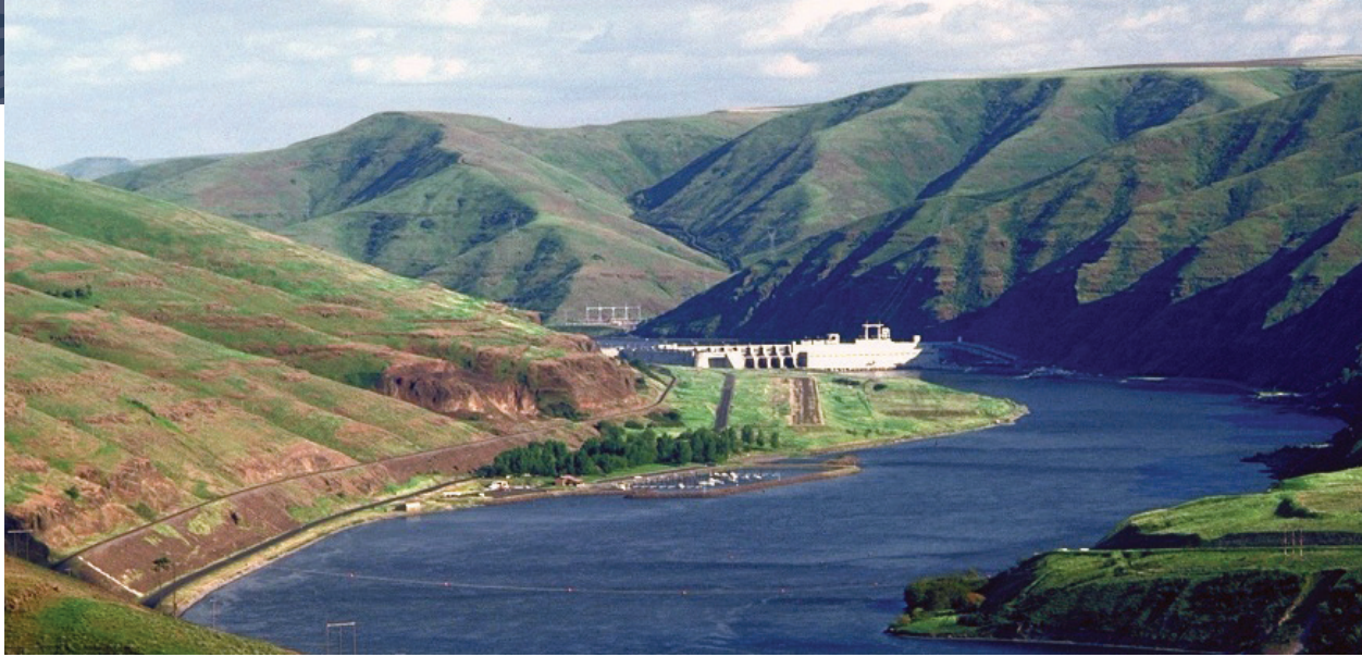
Lower Granite Dam
